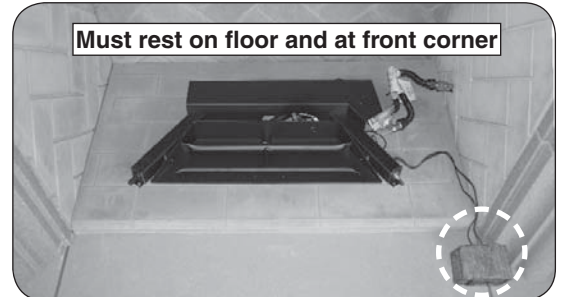
Fig. 19-2 Place heat shield (if applicable)
